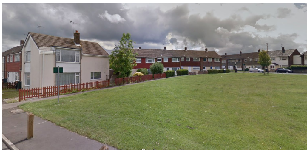
Figure 11: View of 2 Watercress Lane and 32-38 Cross Stile
